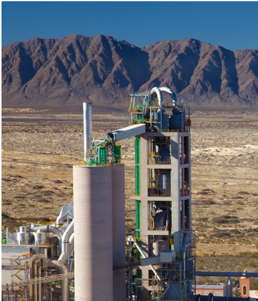
Controlled Burn (a cement plant currently burning TDF)
